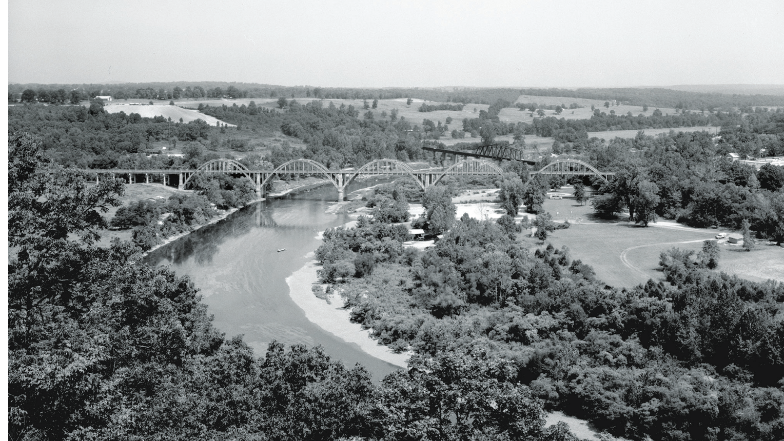
With a length of 1,850 ft, the R.M. Ruthven Bridge was the largest rainbow concrete arch bridge designed by James Barney Marsh.
