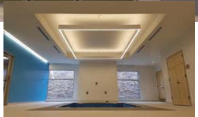
TANGENT UpDown™ • Nemours duPont Pediatrics, Deptford, NJ • Design: Array Architects
