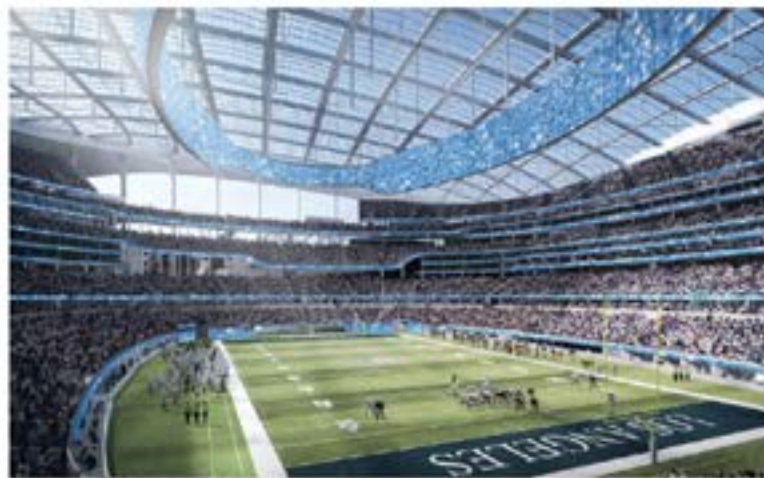
A rendering of the forthcoming Los Angeles NFL Entertainment District Stadium featuring an expansive ETFE roof and ample daylighting on the field of play and in the bowl.
