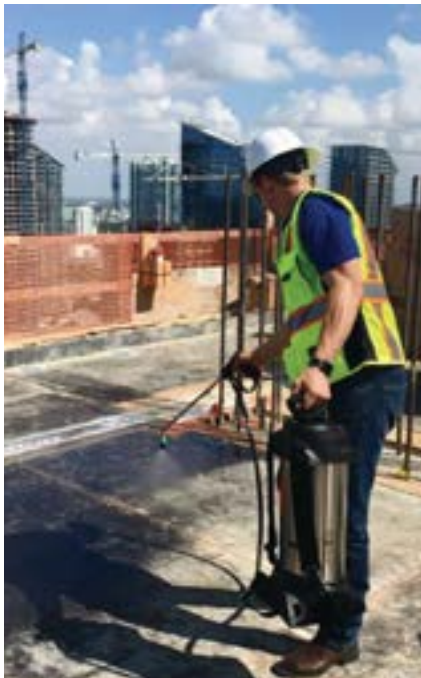
A chemically reactive release agent will give overlaid panels the longest life and should be applied before the first pour. Check with the manufacturer of the forming plywood for more details. PHOTO: NOX-CRETE PRODUCTS GROUP
