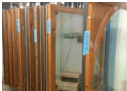
THE MINNESOTA STATE CAPITOL'S NEW WINDOWS NEEDED TO REPLICATE THE HISTORIC WINDOWS, BE ENERGY EFFICIENT AND OPERABLE. TO MATCH THE CAPITOL'S INTERIOR WOOD, 100-PLUS-YEAR-OLD LOGS WERE FOUND IN IDAHO LAKES, MILLED AND STAINED.
