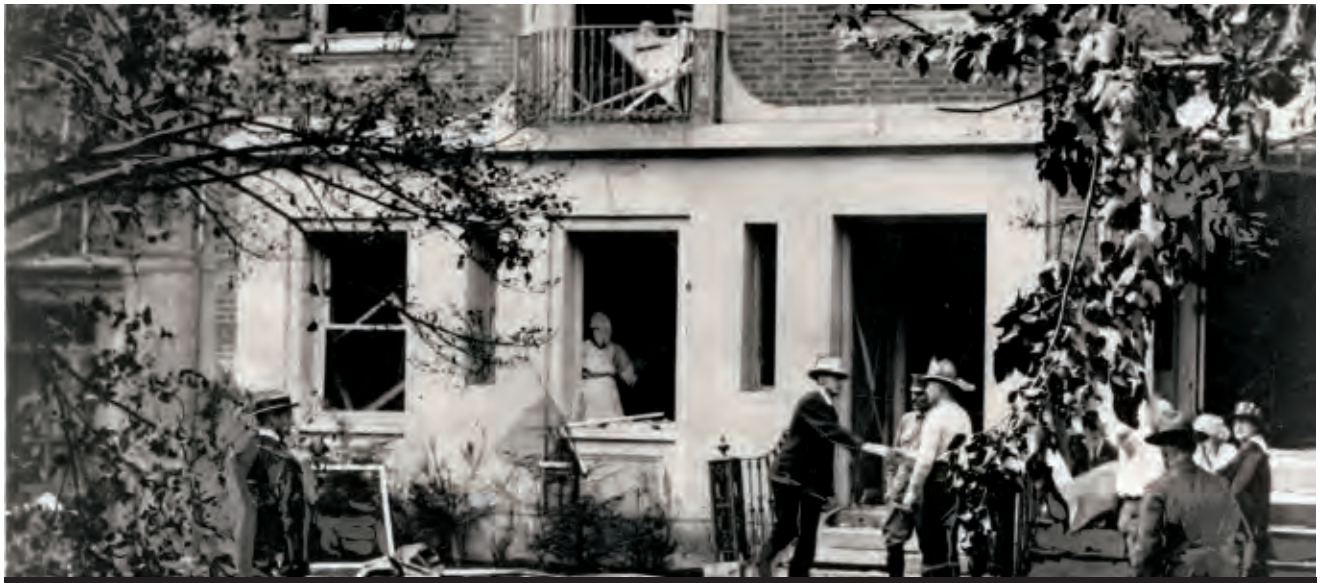
The attorney general's Dupont Circle home was just one damaged in a multicity bomb attack on officials deemed hostile to organized labor.
