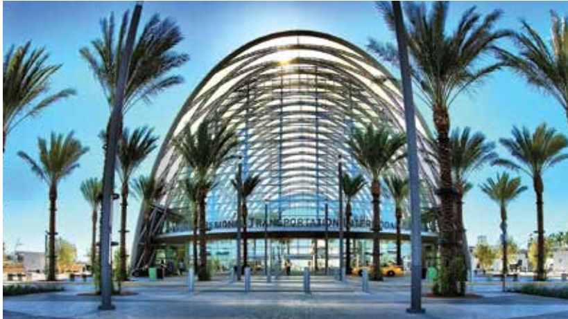
Photo courtesy of Helix Electric
