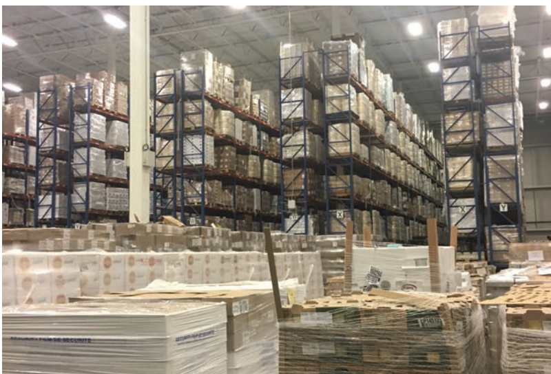
The Seafriigo cold-storage facility in Elizabeth, New Jersey, demonstrates the vertical stacking of products, which can help bring down refrigeration costs.
