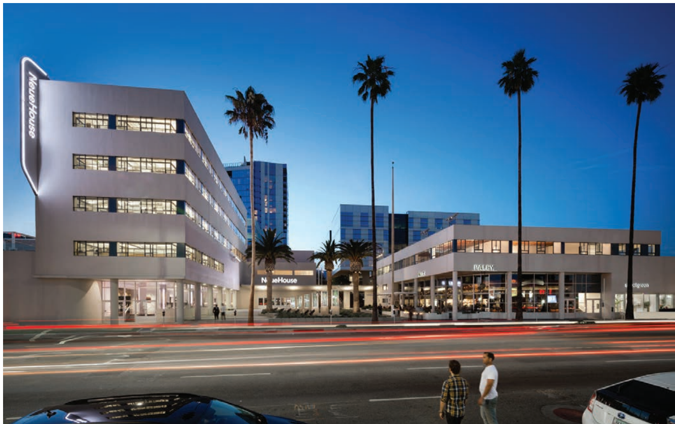
Columbia Square in Hollywood is an adaptive reuse of a complex that was once the West Coast headquarters of television and radio giant CBS.
