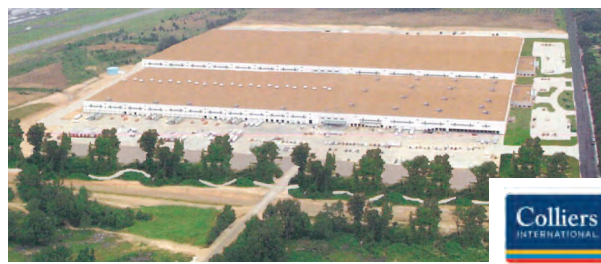
Williams-Sonoma Distribution Center Olive Branch, Mississippi | Disposition | $48 M | 1,060,433 s.f.
