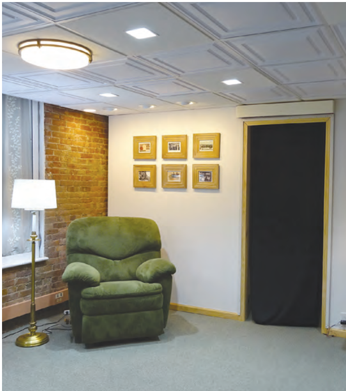
Circadian-friendly lighting strategies may be beneficial for residents of senior facilities. The Lighting Research Center's 24-hour lighting scheme demonstration room provides cycled electric lighting with cool, high light levels during the day and warm, low levels in the evening.
