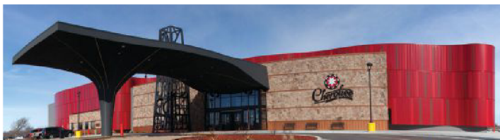
Cherokee Casino Ramona in Ramona, OK Owner: Cherokee Nation Entertainment; Architect: Selser Schaefer Architects; Contractor: RMZ Builders Installer: Abcco Roofing; Profiles: Perforated Flush Panel, Flush Panel, PAC Precision Series HWP, 7.2 Panel, 7/8" Corrugated, Flat Sheet; Colors: Colonial Red, custom Bright Red, Copper Penny, Slate Gray
