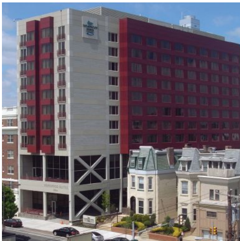
Hospitality buildings such as this Homewood Suites by Hilton in Philadelphia, Pennsylvania often make extensive use of structural steel.
