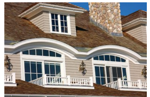
Short lengths, around windows for example, can and should be built with tight joints. Photo courtesy of VERSATEX Trimboard
