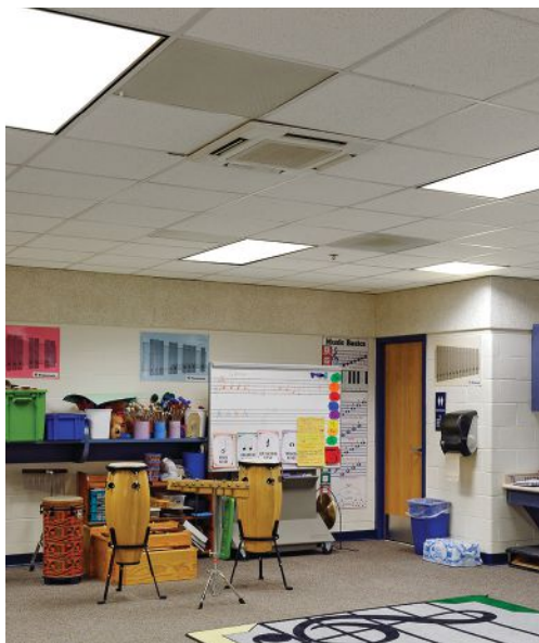
Independent zoning in the modular VRF systems means one zone can be serviced without taking the system offline or disrupting another zone.
