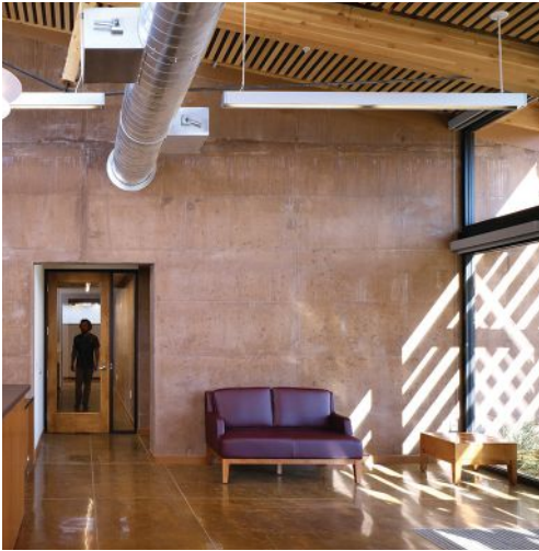
Wood factors prominently in the Ranger Station's aesthetic, from furnishings and accents to structural design.
