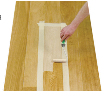
With hardwax oil finishes, you can tape, sand and refinish for an easy spot repair.
