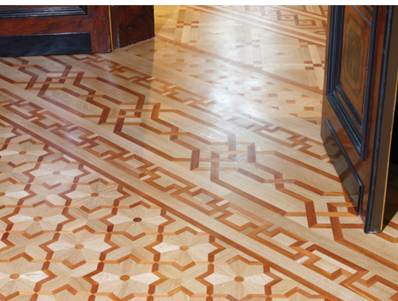
Top: The original parquet floors of the M-Museum in the process of being sketched for reproduction. Bottom: The reproduction.
