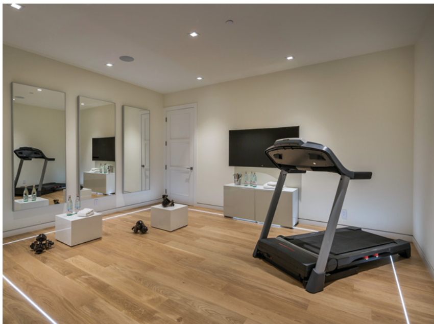
This European white oak floor installed by San Francisco-based Area Floor Works appears to have a standard aluminum feature strip (top)—until the LED lights inlaid with the aluminum are turned on (bottom).
