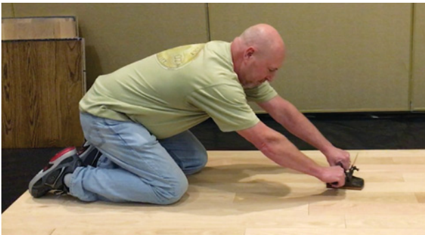
Top left, Vance Hough [at right] and his nephew, Walter Cornwell, with a wood flooring bumper that was used by Hough’s father to scrape floors. Bottom, Cornwell demonstrates how the bumper was used.
