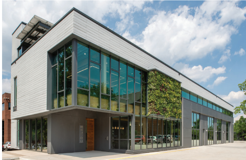
Photo by John Cole, Courtesy of HITT Contracting
