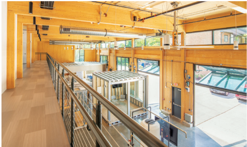
Photo by John Cole, Courtesy of HITT Contracting
