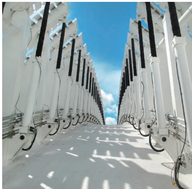
A series of hydraulic cylinders were used to pivot 47 aluminum louvers on each side of the Innovation, Science and Technology Building. Each hydraulic cylinder is fitted with electronically controlled proportional valves and an electronic position feedback transducer that communicates the position of the cylinder and louver to a programmable logic controller.
