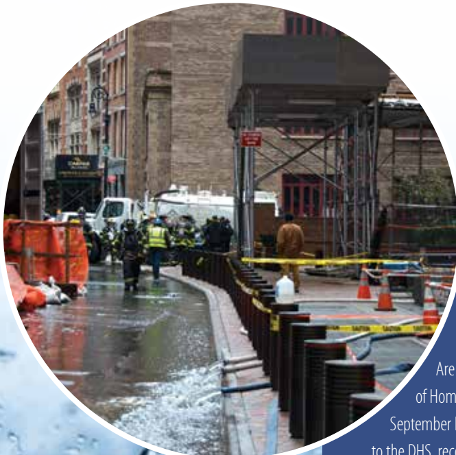
Work crews use pumps to extract water from flooded basements.
