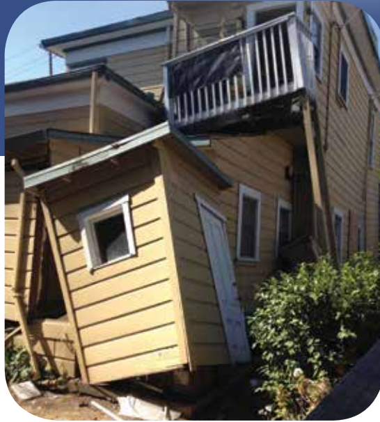
The Napa, California, earthquake in 2014 left 70,000 residents without electrical power. Photo courtesy of the City of Sebastopol, California
