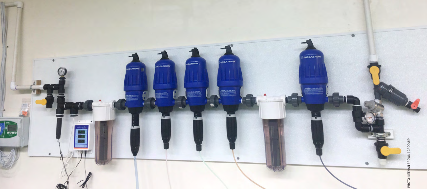
The Dosatron pumps Good Meds installed inject fertilizer into the water lines based on a dial setting. The mixture flows to drippers located at each plant. The system ensures the precise amount of nutrients are being dispersed at a set gallon-per-minute rate.
